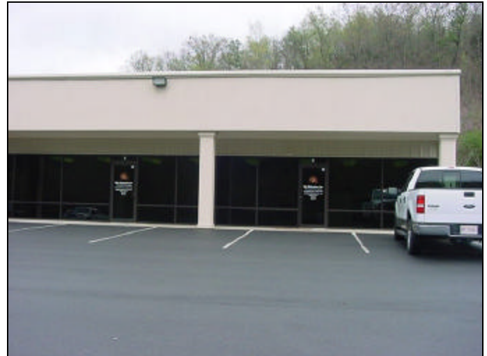
Epic Dalton Warehouse , 1223 Coronet Drive
